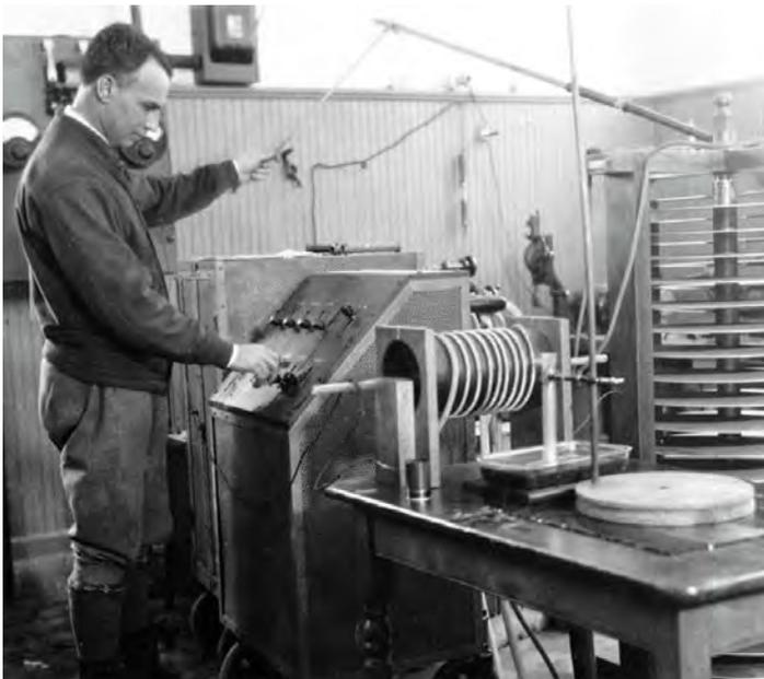
**Figure 4.** Alfred Lee Loomis (1887–1975) in the laboratories at Tower House (Tuxedo Park, NY). Einstein dubbed it the “palace of science.” The apparatus is the high-voltage oscillator used to drive a quartz piezoelectric transducer to produce intense ultrasound. Photo courtesy of the Smithsonian Institution Archives, image #SIA2008-5428.
